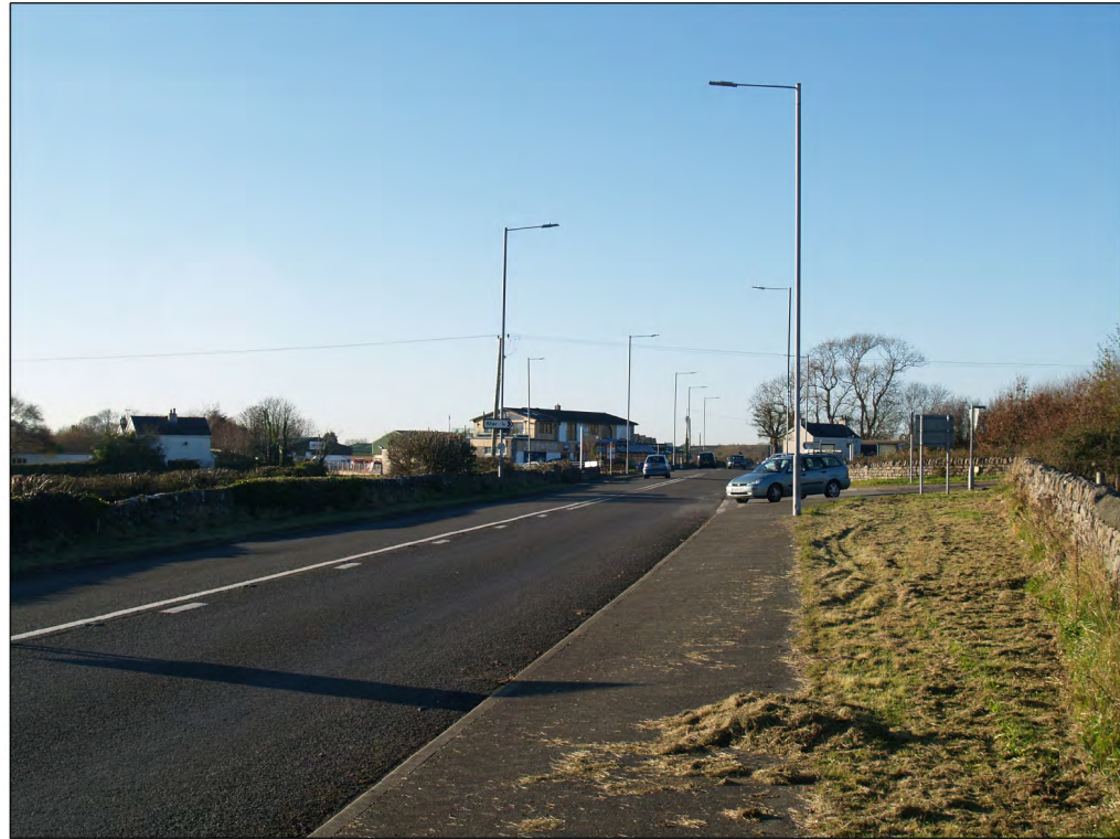
Photograph looking west toward the Star junction with a minor road which crosses over the A55
